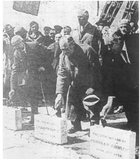
Lympstone dignitaries Garbutt Knott, Norman Jenkins and Major Barton Aitken lay the foundation stones for the restored boat shelter.
